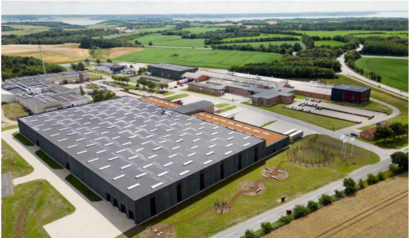
SKOV Headquarter, R&D, Test Center & Production. Glyngøre.
